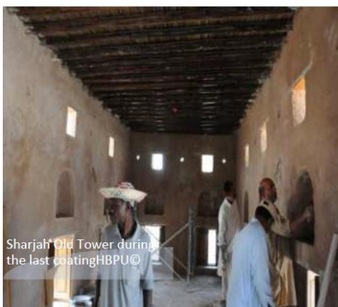
Figure 9: pictures of applying some of the new mortar in some Sharjah restoration projects
