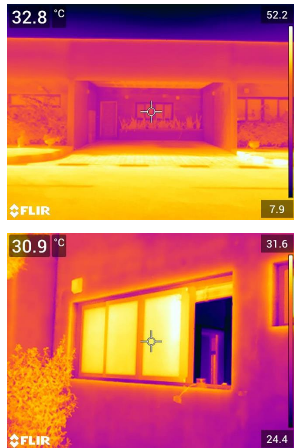
Figure 1: Thermal Image of the Villa from the Entrance
