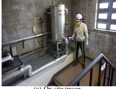
(a) On-site image.
