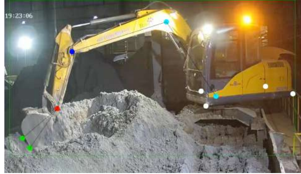
Figure 7. Excavator pose estimation result.
