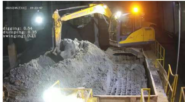
Figure 8. Excavators long video action detection result.
